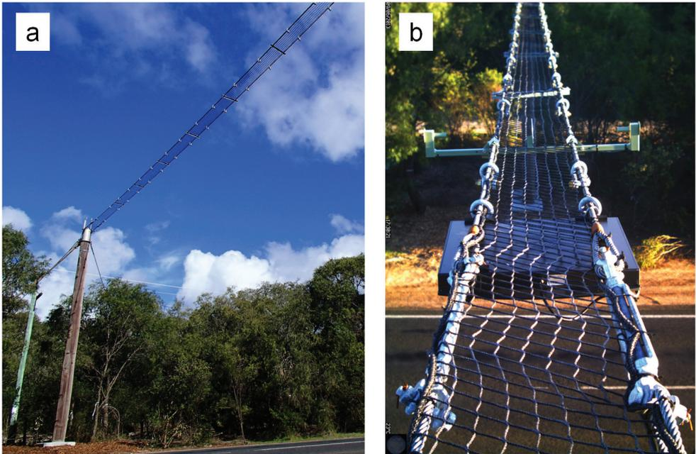
**Figure 2.** A rope bridge installed on Caves Road near Busselton, Western Australia. **a** Two stay wires and a rope extending from the pole of a rope bridge to nearby trees on South side of Caves Road **b** Close up of the bridge showing one of the sensors and microchip reader on the North side (taken by an infrared camera on the bridge).
