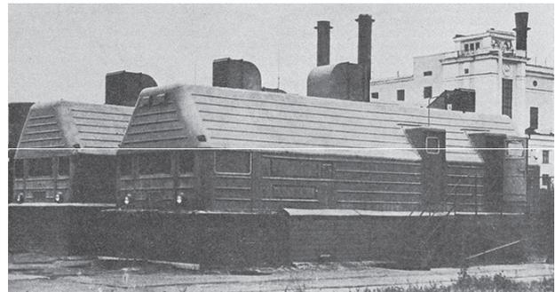
**Figure 2.** View of the self-propelled vehicles with a control panel and a turbogenerator. The tracks are closed for winterizing (Sinev et al. 1964).
