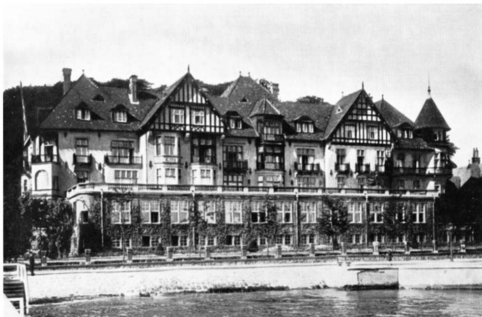
Fig. 2. Building of the Kiel Institute of World Economics 1920–1943.
