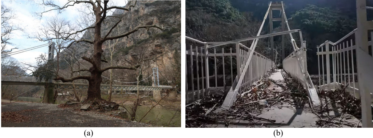
FIGURE 3. Tempi bridge located in Agia Paraskevi church on the Pinios river banks: Before (a) and after (b) Daniel's storm flood disasters.
