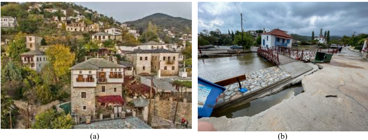
FIGURE 2. Traditional settlements in Pelion region: Before (a) and after (b) Daniel's storm disasters.
