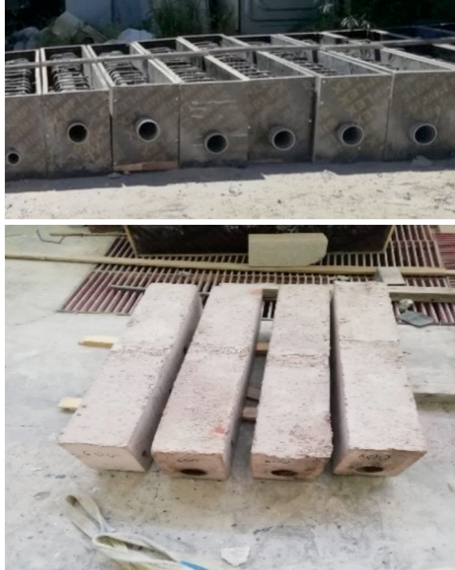
FIGURE 4. Preparation process of the beams.
